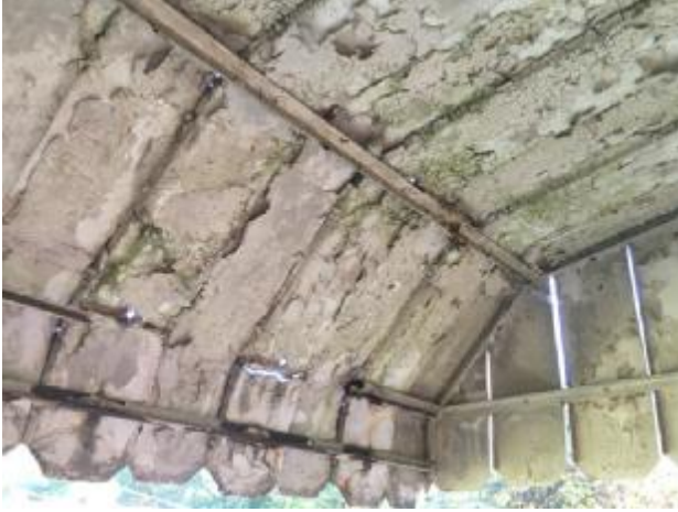
Front porch awning
