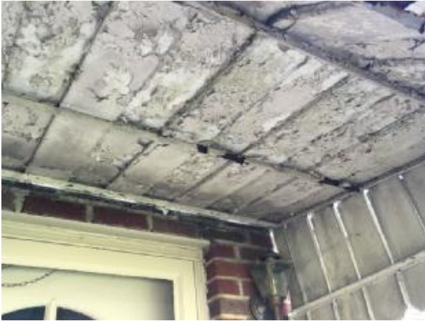
Front porch awning
